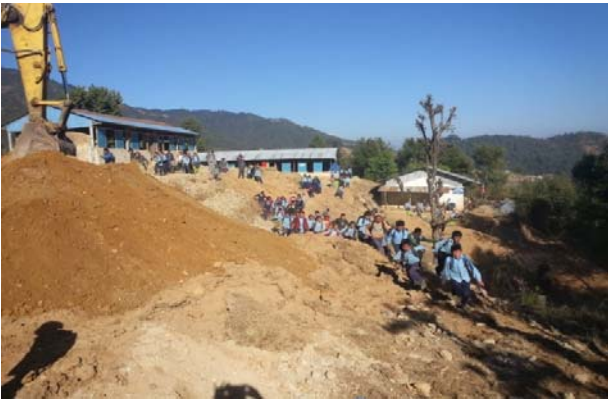
Excavator leveling the ground
