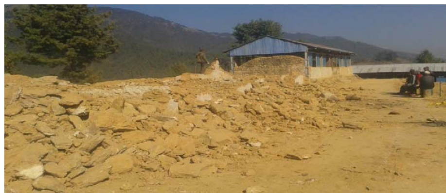
Damaging old building for reconstruction
