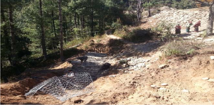
Wall work for sloppy land
