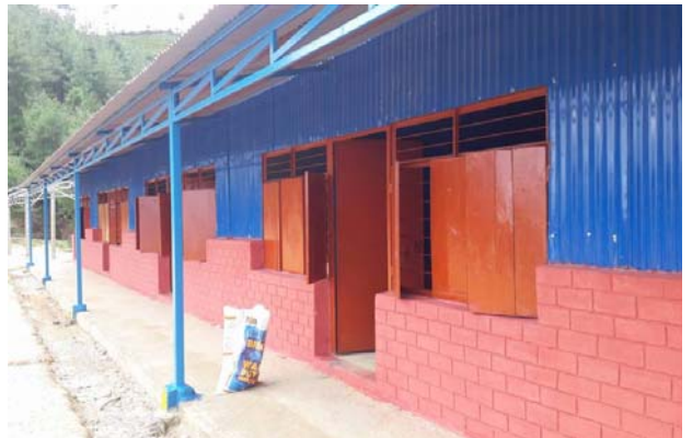
Completed reconstruction School building
