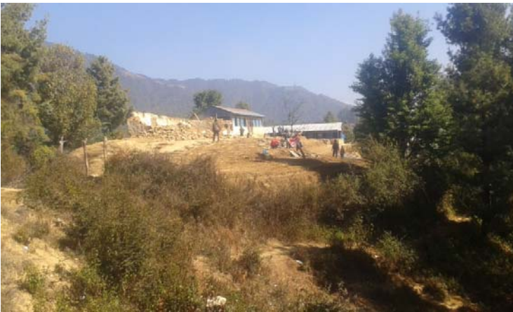
Badly damaged School Building by earthquake in April 25, 26 and May
